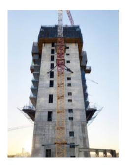
They also used our T-type safety net system, a system for arresting people and objects from falling. This system consists of a safety net attached on brackets for horizontal use.
