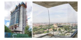
For the vertical protection of Caleido's personnel, in Visornets we supplied U-type safety net systems that acted as a vertical enclosure. In this way, the movements of the equipment were restricted, preventing falls at different levels.
