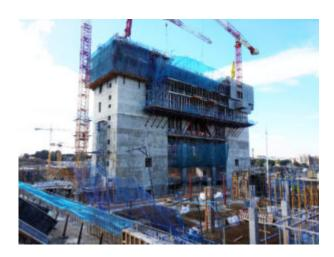
V-type nets are a system consisting of a safety net with a border rope attached to metal gallows by means of tying ropes. This way the fall of people and objects is limited from a maximum permitted height of 6 meters and recommended 3 meters.
