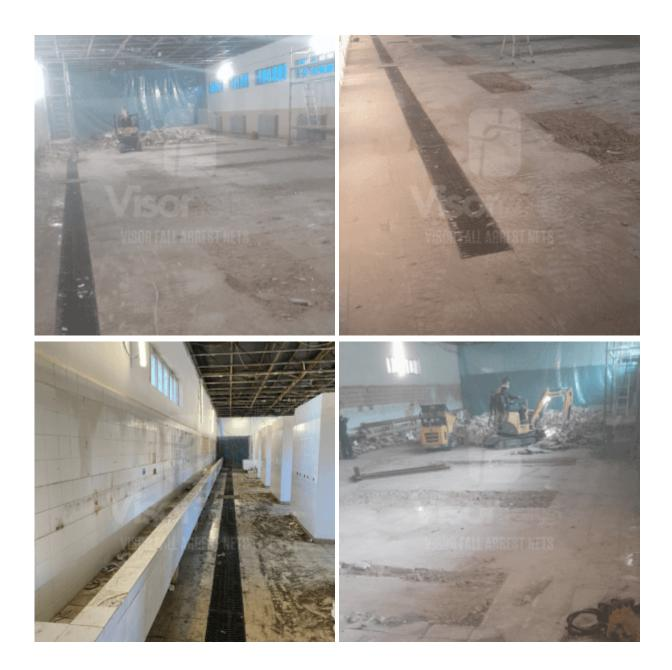
As can be seen in the result, the work area has been completely isolated and clean, which makes this Safety Net + plastic membrane a fully compatible system that achieves the desired result.
