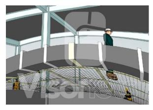
the inclination of the installed net will not be more than 20° (or maximum slope of 36,4%),
