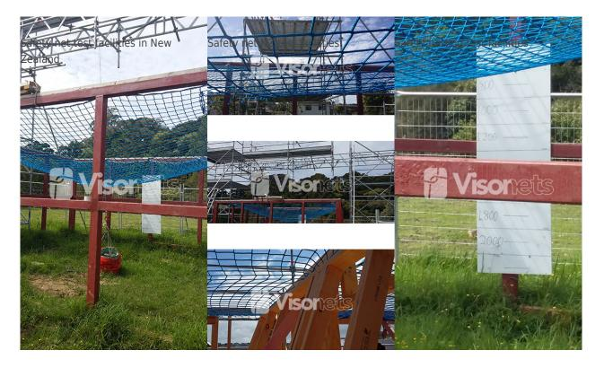
As the vast majority of the **safety** nets installed in New Zealand are for residential houses, better known as **residential safety nets**, they have developed their own anchorage systems, being the nets directly installed to the wooden beams.
